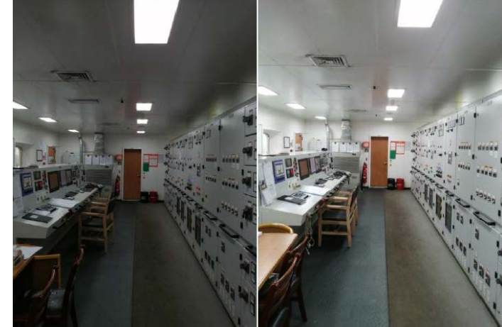
Engine Control Room - Before and after LED light installation photos
